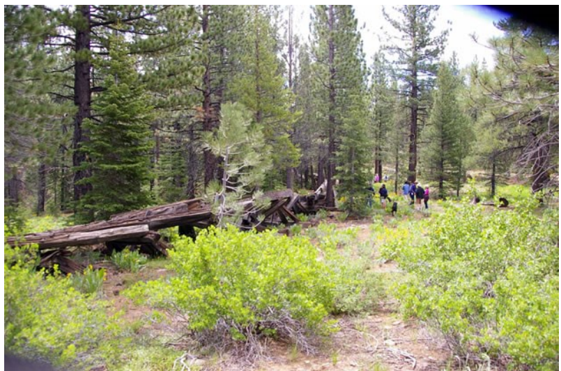
Remnants of a trestle in the forest north of Truckee (pc TDRS)
